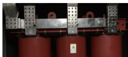
Joint point of transformer extending busbar temp. detection
