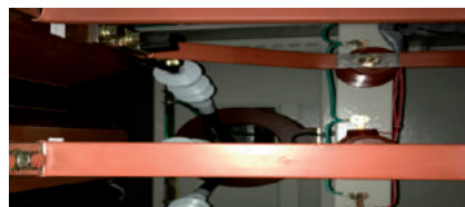
Temp. detection between cable and busbar joint point
