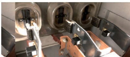
VCB claw type contactor temp. detection
