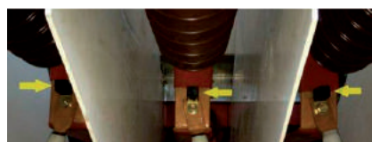
Temp. detection between cable and busbar joint point
