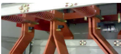
Main busbar temp. detection
